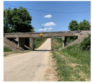
Figure 18: S Browns Mill Rd Crossing – East of Freeport. Deterioration of concrete piers is visible.
