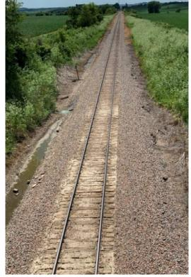
Figure 16: Photo taken from the E Roberts Rd Crossing depicting track with fouled ballast and a ditch with standing water
