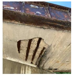
Figure 17: E Yellow Creek Rd crossing – East of Freeport. Concrete spalling and rusting of the steel girder is evident.
