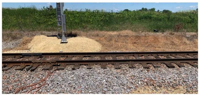
Figure 15: Photo taken near the Alworth Rd. crossing from an adjacent road depicting split ties
