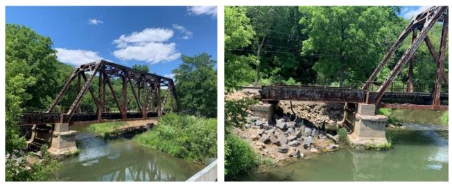
Figure 19 & Figure 20: One of several bridges of the East Fork Galena River east of Galena. Deterioration of the concrete pier and rusting of the steel members is visible.
